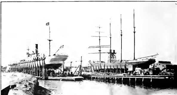
Marine Railway at the Alameda plant of the General Engineering Company.
